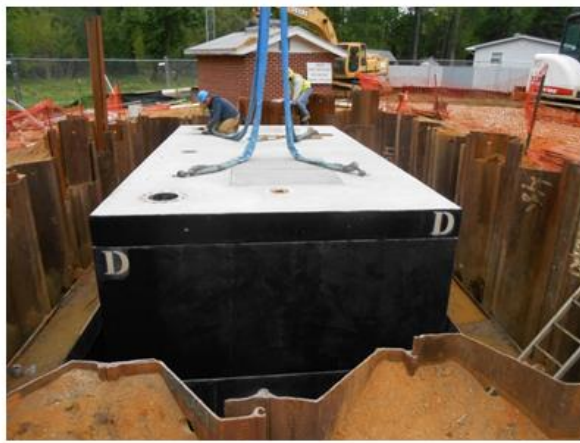
Lynn Drive Waste Water Pump Station Project: New Wet Well Storage Vault in Place
