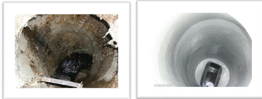
Before and after photos of a repaired and sealed manhole in MetCom sewer system.
