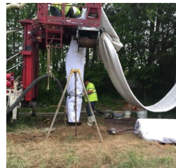
Contractors installing a resin – impregnated felt liner into large gravity sewer line.
