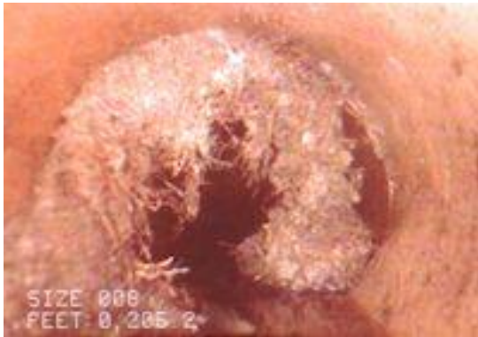
Photos of both root intrusion (left) into sewer lines and the build-up of grease on the interior of sewer lines (above).
