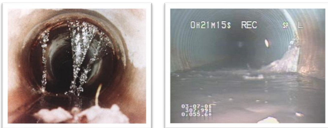
Pictures (above) show infiltration that can enter the sanitary sewer system through cracks and other defects, increasing flows at pumping stations and treatment facilities.
