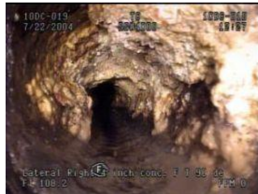
Photos of both root intrusion (left) into sewer lines and the build-up of grease on the interior of sewer lines (above).
